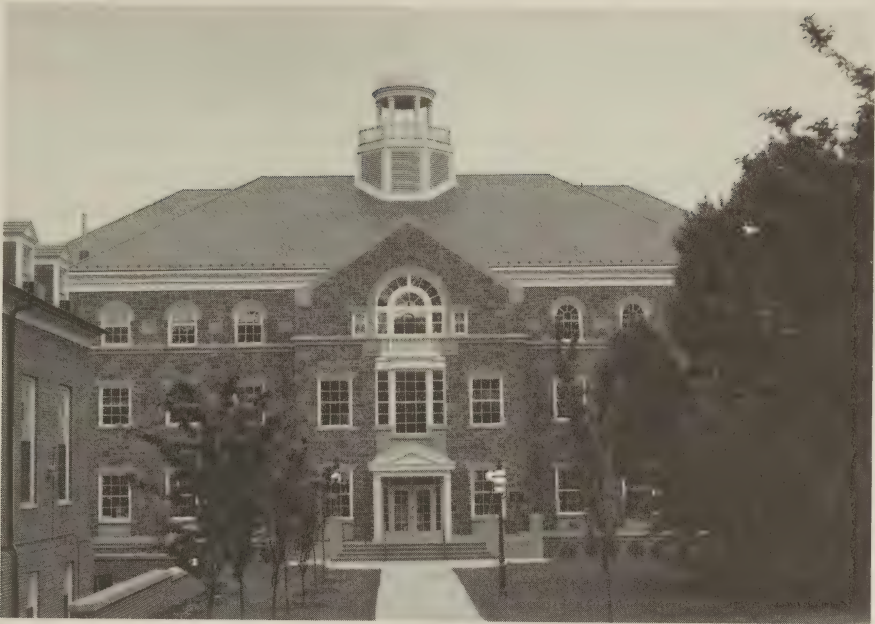
Templeton Hall — Completed 1989
